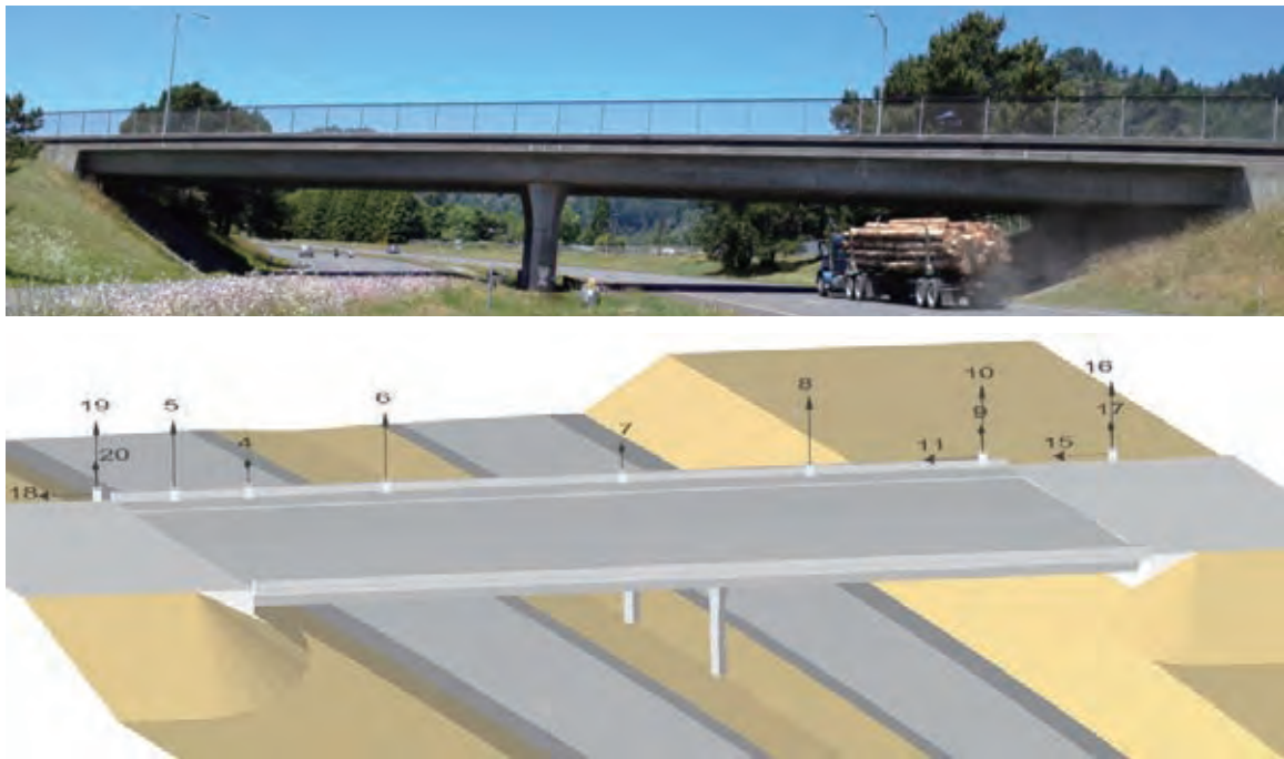
Figure 3. The Painter Street Overpass (top) and its seismic instrumentation (bottom).
