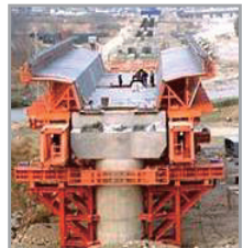
Construction view of Sangchon Br. using MSS
