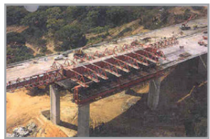
A construction stage view of MSS
