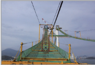
Pylon & catwalk of Kwangan Grand Br.
