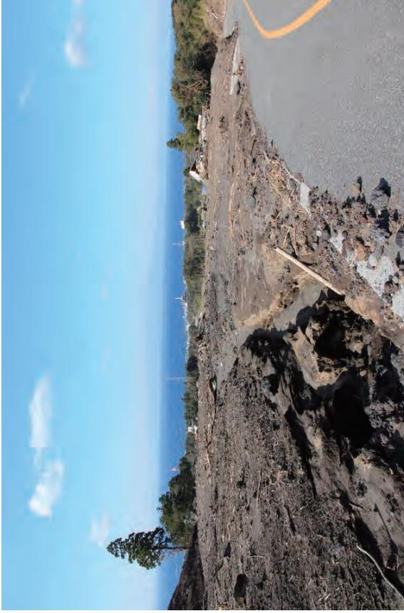
Rainfall induced slope failure
