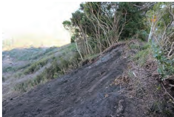
Very thin failed layer
