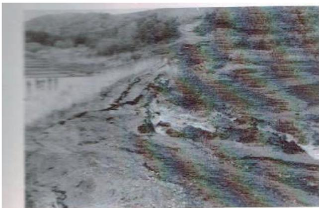
Fig. 13. The damage to the Yamanaka dam caused by the 1968 Tokachi-Oki earthquake.
