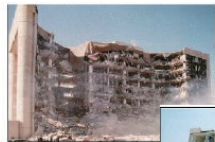
Figure 1.1 Murray Building, Oklahoma City
