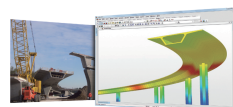
Lee Roy Selmon Flyovers (U.S.A.) Balanced Cantilever Bridge with Approx. 90 Degrees in Curvature
